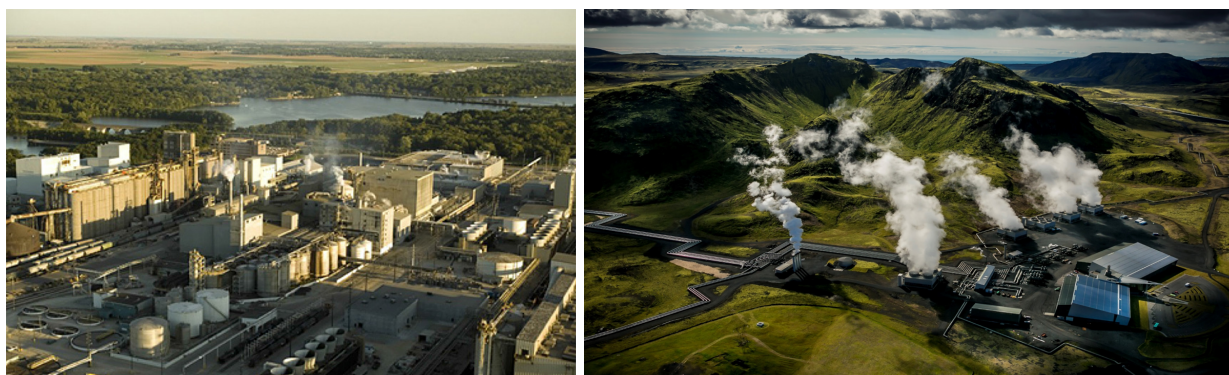
Figure 3 | Existing Sequestration efforts. Left: The Archer Daniels Midland project can store roughly 1 million tons of CO 2 per year in the Mt. Simon Sandstone, Illinois Basin, which has an estimated storage potential of over 250 million tons of CO 2 per year ( link ). Right: The site of the CarbFix project in Iceland, which has buried 200 tons of CO 2 by pumping carbonated water into basalt at $25/ton.
