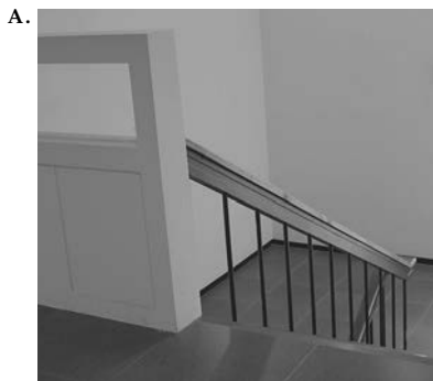
FIGURE 1.5. Accidental Affordances Can Become Strong Signifiers. This wall, at the Industrial Design department of KAIST, in Korea, provides an anti-affordance, preventing people from falling down the stair shaft. Its top is flat, an accidental by-product of the design. But flat surfaces afford support, and as soon as one person discovers it can be used to dispose of empty drink containers, the discarded container becomes a signifier, telling others that it is permissible to discard their items there. (Photographs by the author.)
