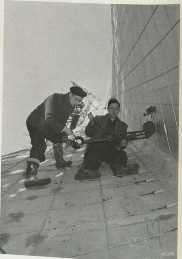
Fig. 11. Tensioning a prestressing wire with the "Strabed" jack. The tensioning force is read on a dynamometer.
