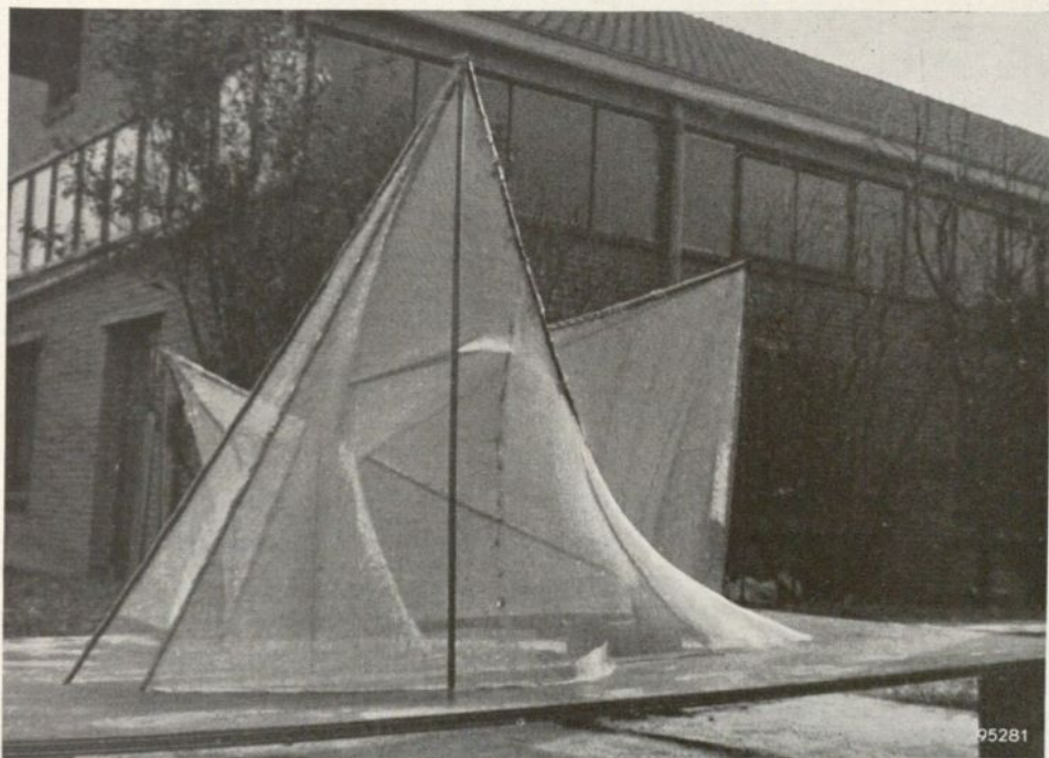
Fig. 1. Framework of tubes and wire-gauze for making the plaster model of Philips pavilion, scale 1 : 25 (T.N.O. Institute, Rijswijk, Netherlands).
