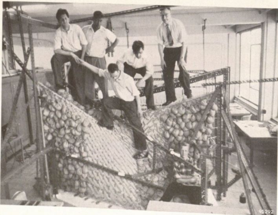
Fig. 14. The plywood model severely overloaded.
