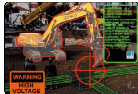
Figure 6-3. Locating utilities could be a specialized application of location linked information systems. Visualized is WorldBoard’s concept of how this might work.
