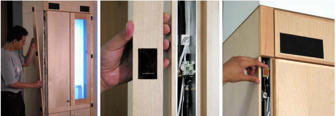
Figure 8. PlaceLab interior testing one aspect of Open Source Building: Integrated Interior Infill (I3) components with sensing and addressable lighting infrastructure. Shown are hinged, accessible sensor bus raceways. All cabinets use the same embedded connections and technologies, simplifying installation and increasing flexibility. The facility contains hundreds of modular sensors.
